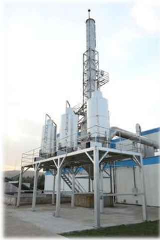
Figure 6 Chimney of Incineration plant
